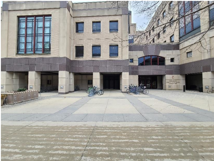
North entrance with bike parking.
